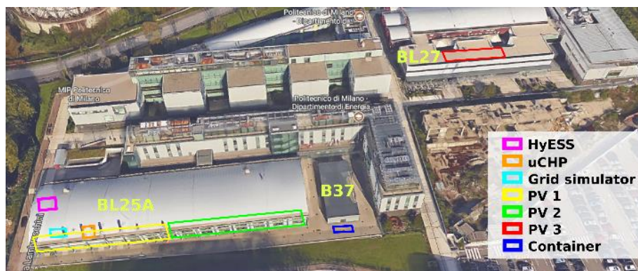
Figure 27: Pilot 4a demonstration site
