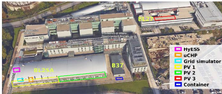
Figure 40: Pilot 4a Demonstration Site
